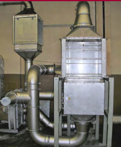
Photos left: : Catalytic exhaust system, individually designed for process- specific exhaust gas quantities and components
